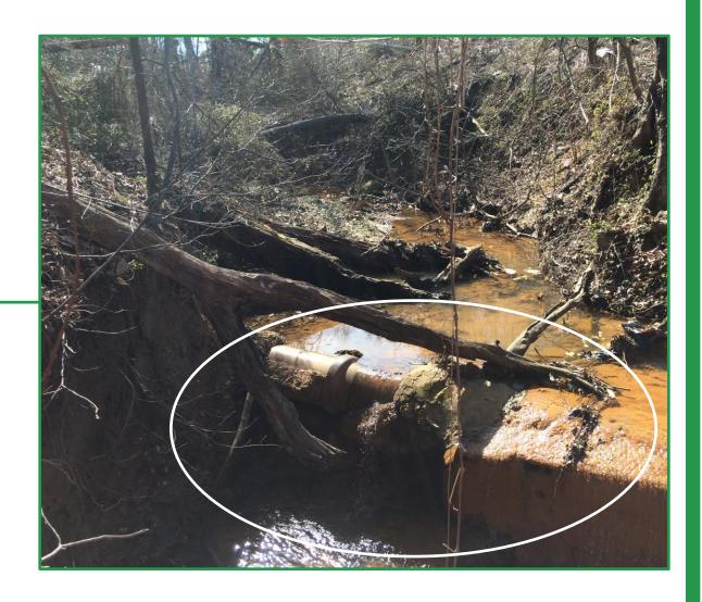
Active streambank erosion and channel incision are occurring within the stream segment.
