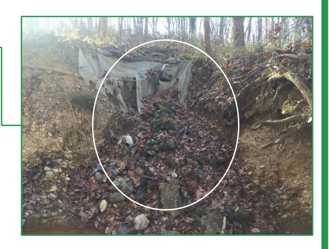
Active streambank erosion and channel incision are occurring within the stream segment.
