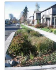
D. Sidewalk Bioretention Planter
