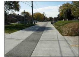
B. Permeable Concrete Alley
