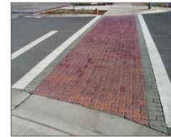
A. Permeable Paver Cross Walk
