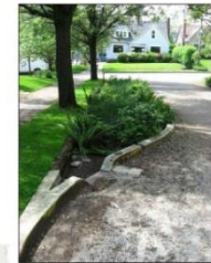
E. Curb Extension Bioretention
