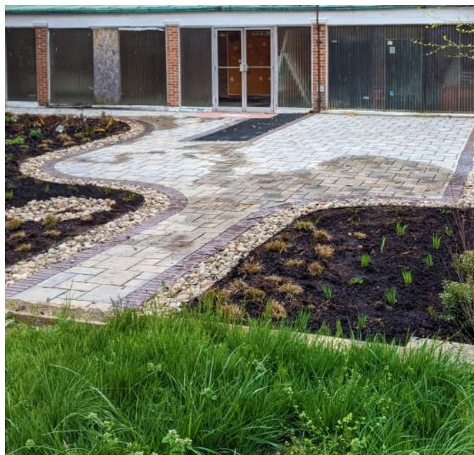
Figure 6 (left) and Figure 7 (right): A rain garden and bioretention installation at two RiverSmart Communities project sites in Ward 2.
