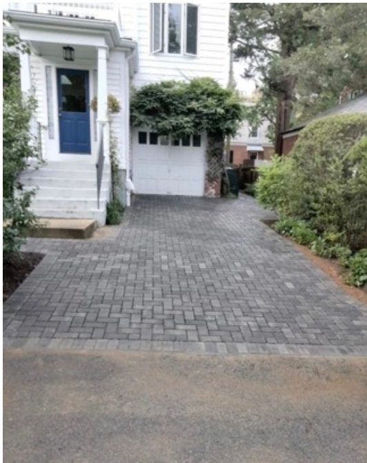
Figure 2 (left) and Figure 3 (right) : RiverSmart Homes permeable paver installation at two homes in Ward 3.
