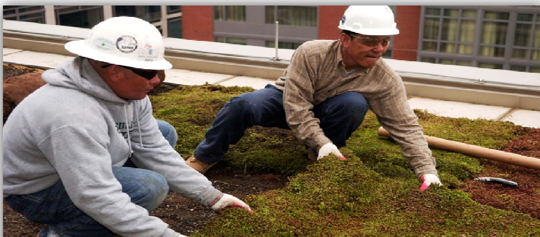
Greening OUR HOUSE: Workers installing vegetated sedum carpet on retrofitted roof at 1200 First Street, NE
