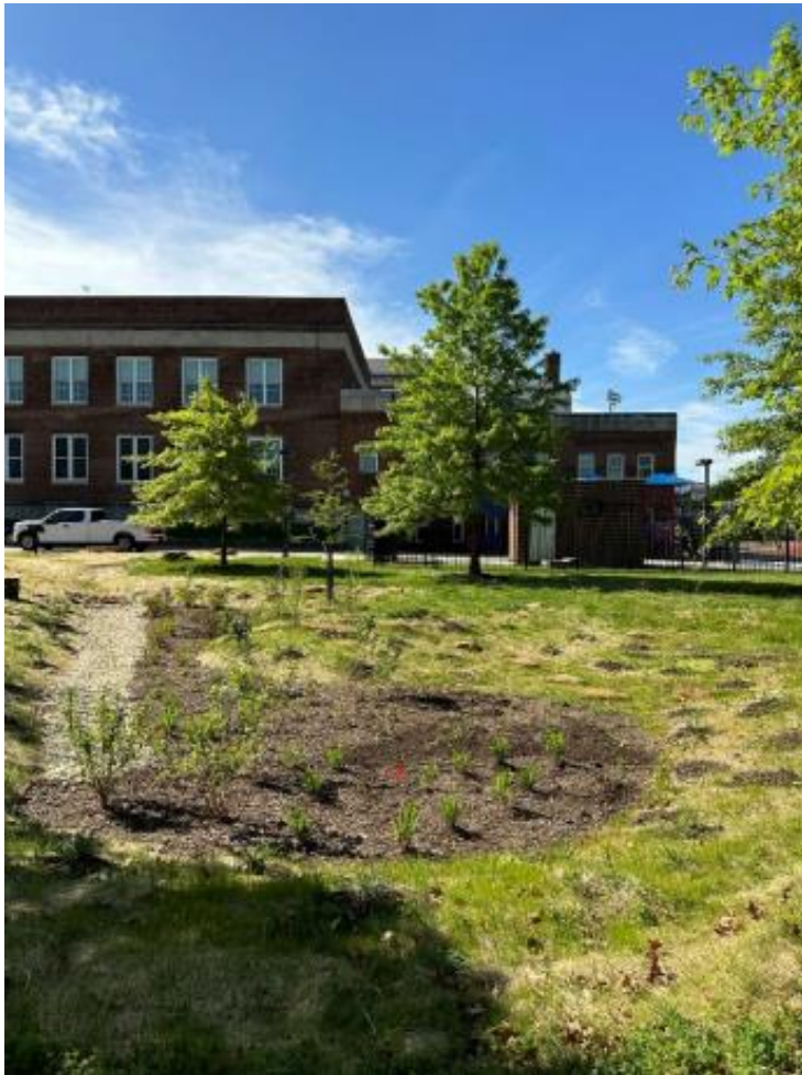
Figure 7 – Bioretention completed at Anacostia High School
