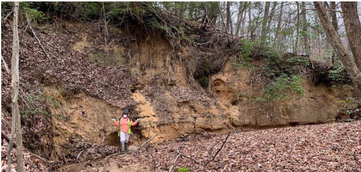
Figure 4 – Severe erosion along Fort Dupont Creek
