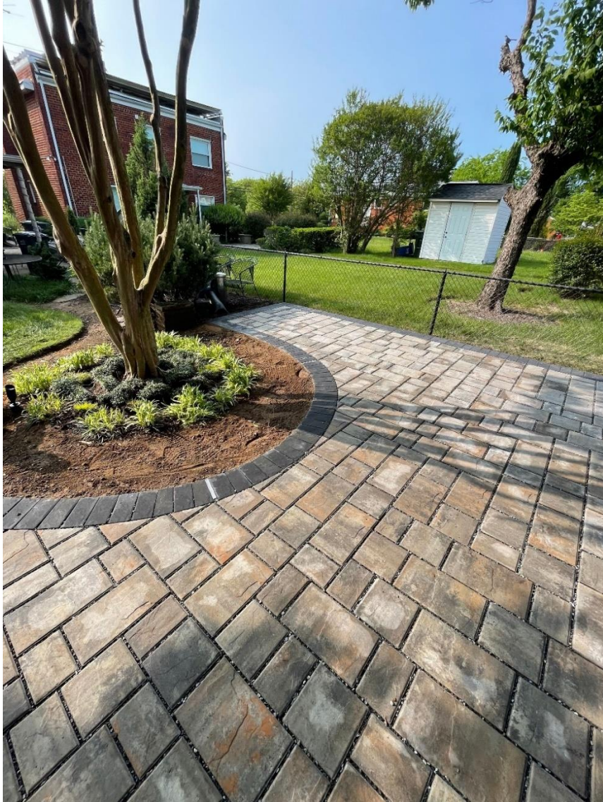
Figure 10 – Residential permeable paver installation
