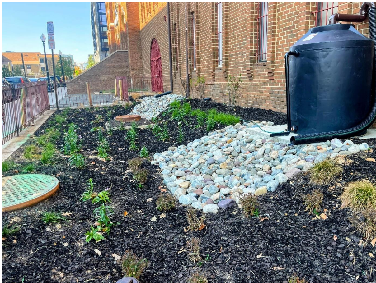
Figure 9 – Cisterns and rain garden at Mount Airy Baptist Church
