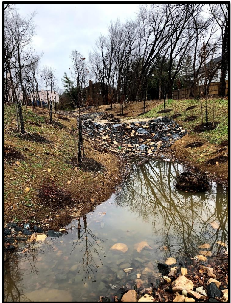
Figure 3 – Congress Heights Stream Restoration
