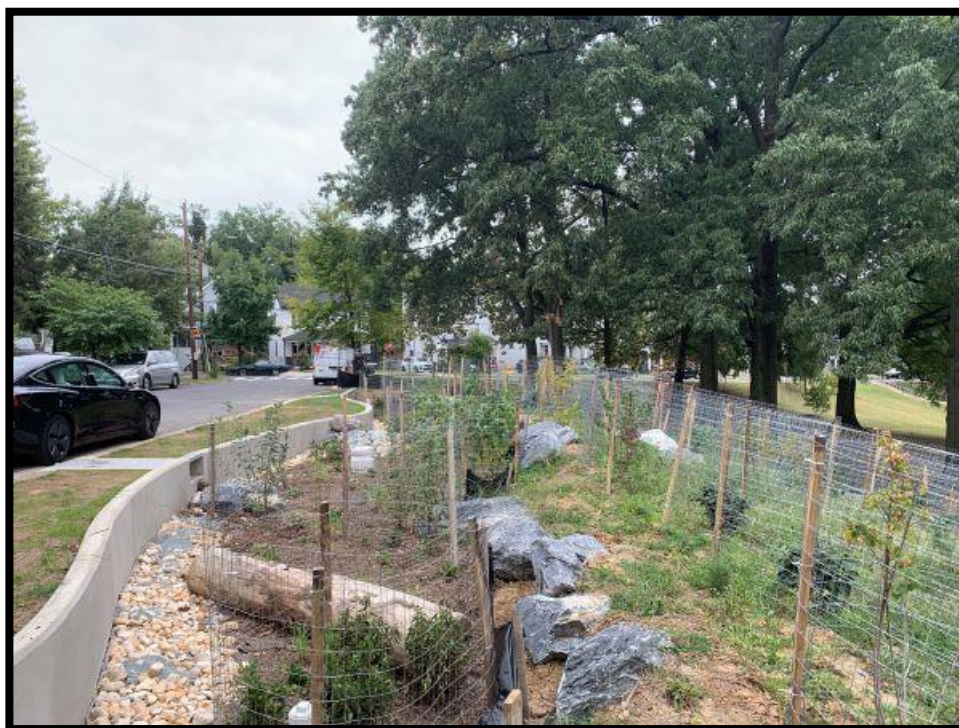
Figure 6 – Hamlin Street Bioretention
