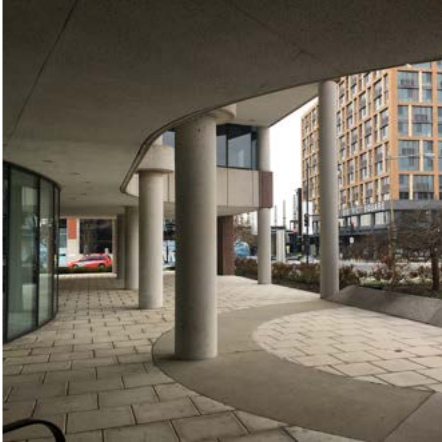
VIEW TOWARDS MAINE AVENUE, UNDER OVERHANG
