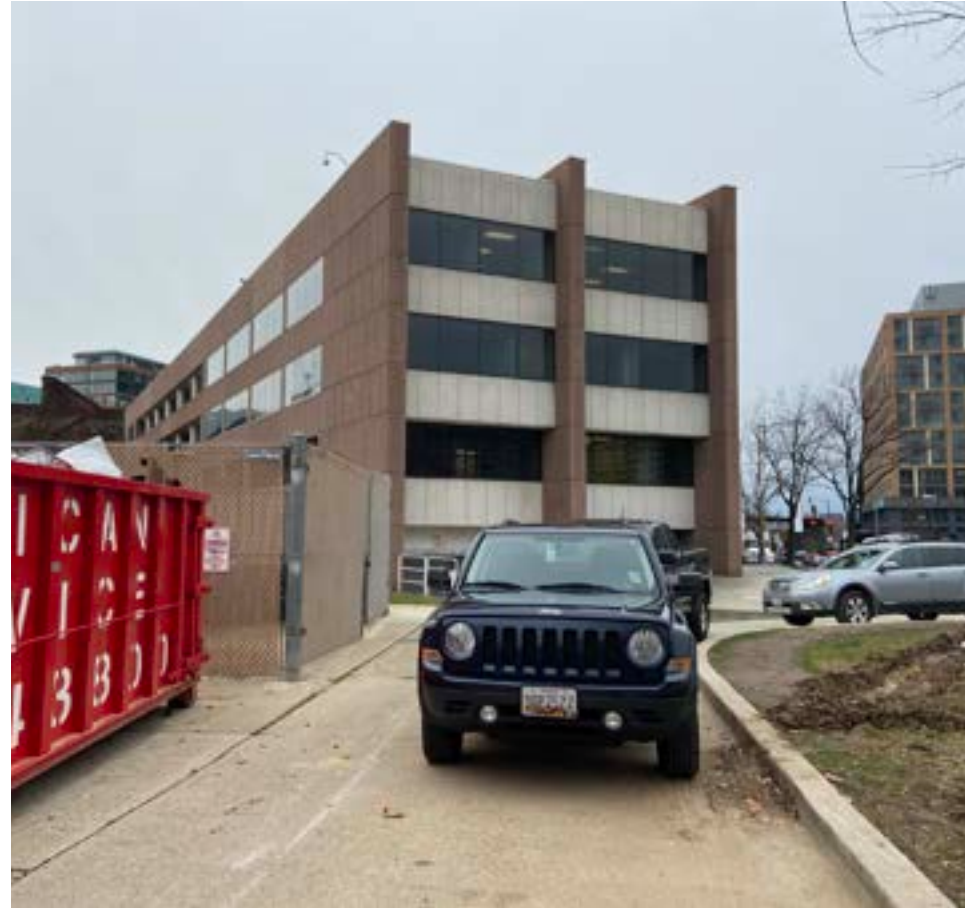
VIEW TOWARD NORTH ELEVATION FROM G STREET, SW
