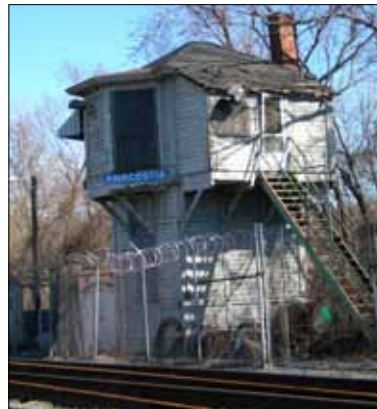
CSX Railway Signal Building, Anacostia Park, demolished, 2008
