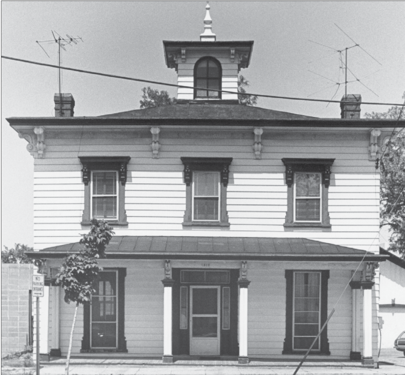
1312 U Street SE, Anacostia Historic District
