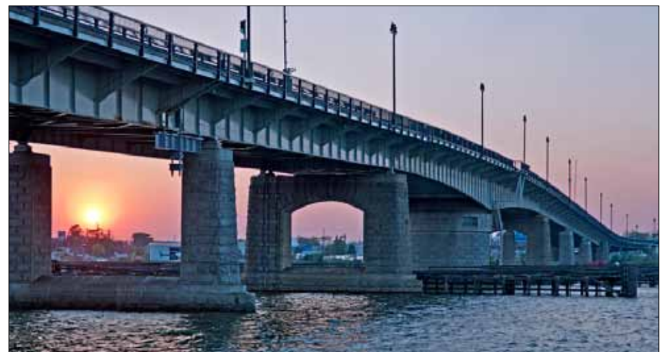
South Capitol Street Bridge Photograph by Brendan Reals
