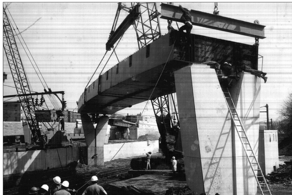
Construction of Interstate 295, 1972 Library of Congress
