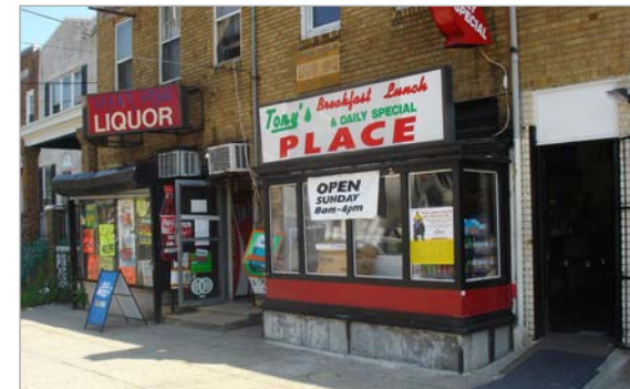
Limited square footage for retail merchandising and concerns about security drive many store owners to fill windows with elements which block views into the retail areas.
